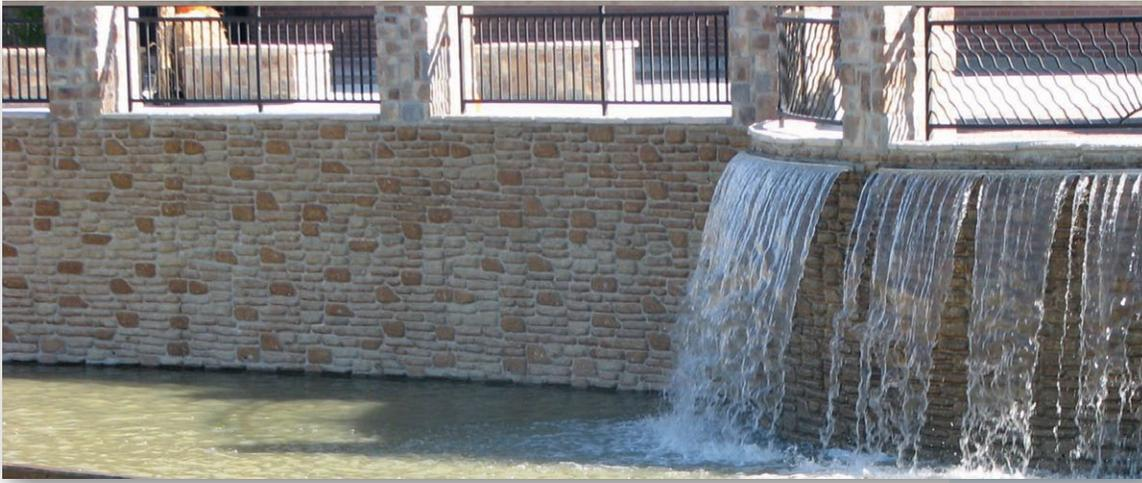
Formliners can be used with any concrete forming system to provide unique designs and economical solutions to forming architectural concrete surfaces.
